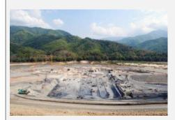
The Xayaburi Hydropower Project consists of a dam of 830 m length and 49 m height, creating a reservoir of 60-90 km in length downstream of Luang Prabang. It is equipped with 10 turbines which will generate 1,260 MW. 95% of the generated electricity will be exported to Thailand. The project is equipped with a navigation lock and various fish passage facilities as well as a system for flushing sediments that get trapped behind the dam.
